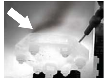
The sniffer is detecting gas but is unable to trace its source, whereas this thermal image shows the leak source clearly on the left.
